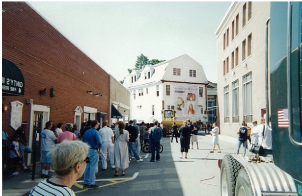
Morrystown, NJ The large structure was moved through the center of Morrystown, NJ. This final street turn was done with just 12 inches of clearance on each side of the building.
