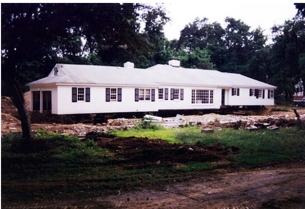
New Haven, CT 120 foot ranch dwelling was moved on the same property to allow for two more houses to be built.
