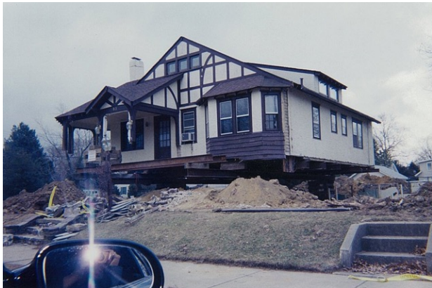
Central Jersey The dwelling was moved 8 feet in order to subdivide the property.
