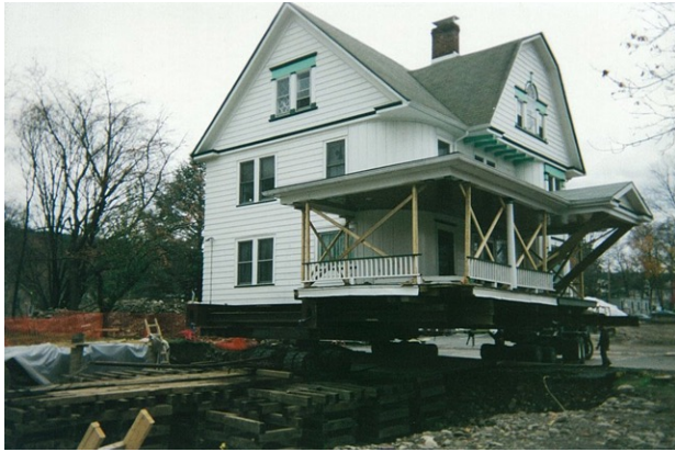
Eastern PA Very old structure complete with plaster walls, was moved so that a church could be built.
