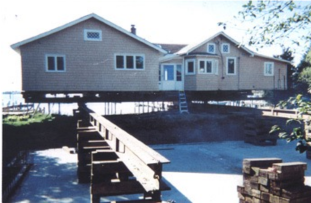
Pricneton, NJ Privately owned structure move on farm property in order to restore the home.
