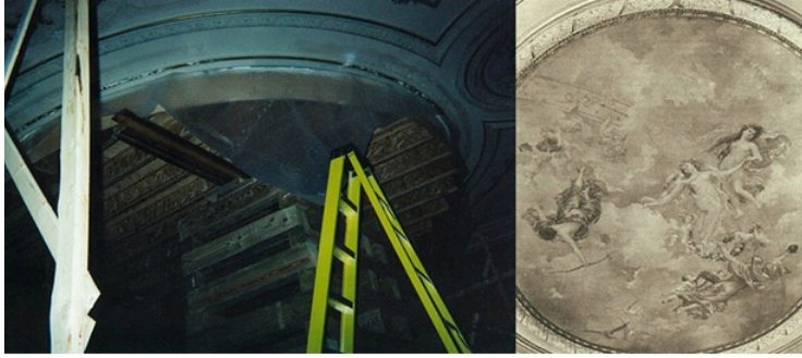
This castle in Pennsylvania has a 100 year old French ceiling painting. W. A. designed and built the equipment to lower the painting from the 20 foot high ceiling. Once the restoration of the painting was complete, we returned it back to its place on the ceiling.
